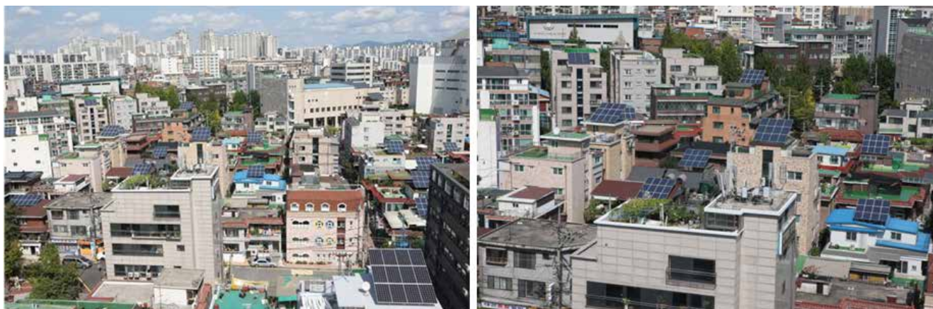
Photo 13.2 High Concentrations of Solar Power Panels Installed on Homes in Shipjaseong Village
