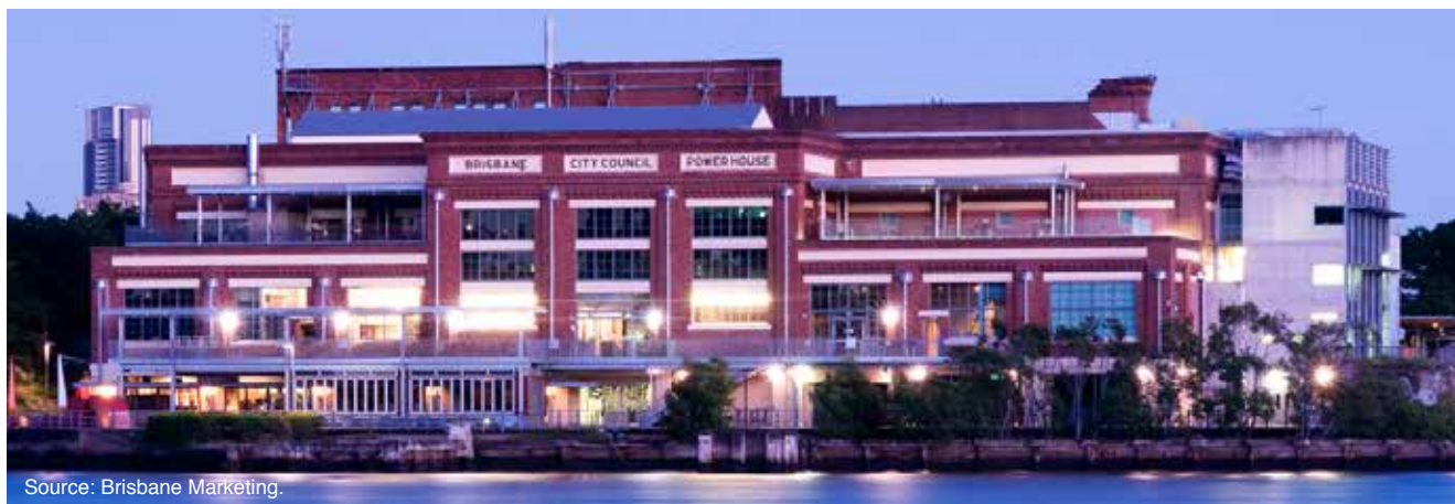
Photo 5.3 Powerhouse Brisbane – From Power Station to Arts and Cultural Facility
