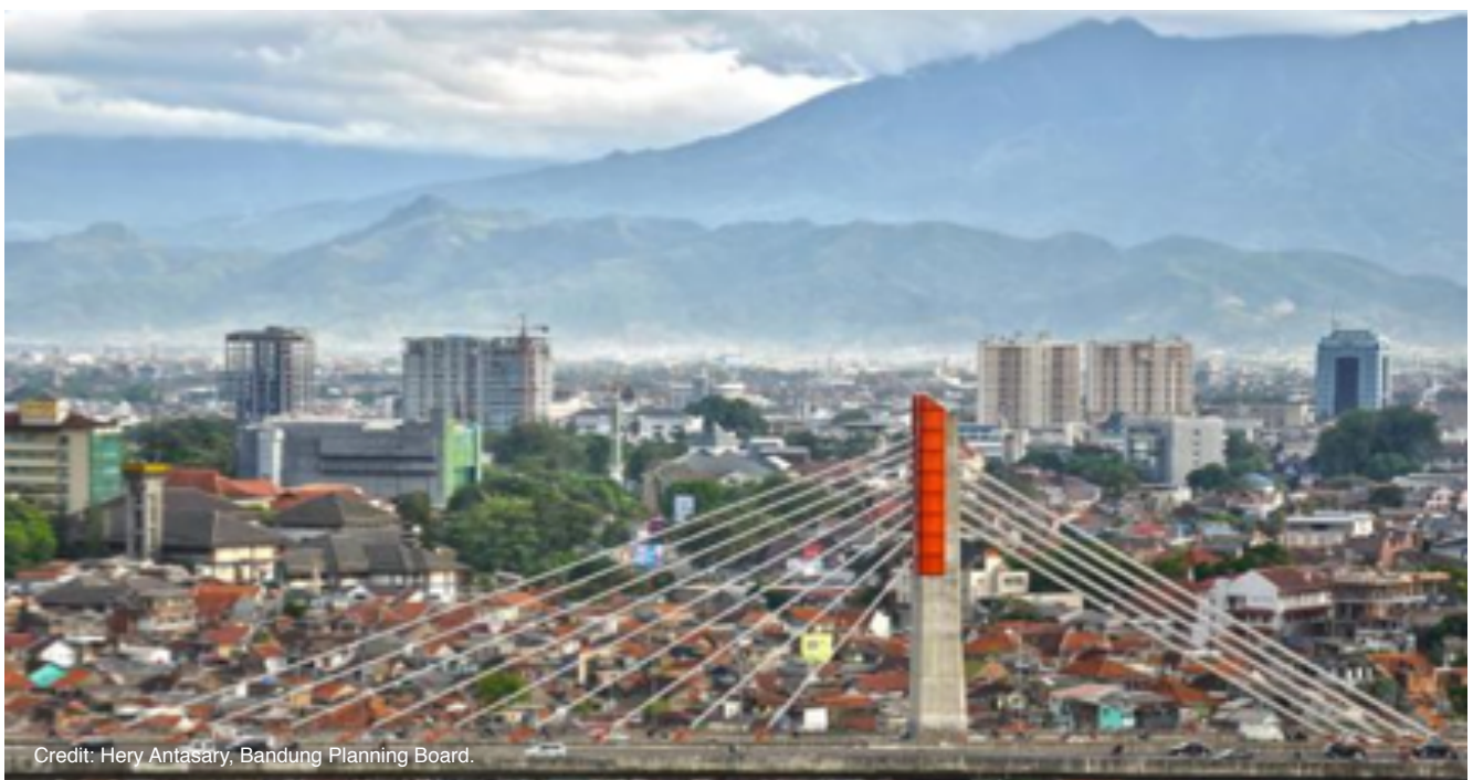
Photo 3.1 Pasupati Bridge, Bandung City
